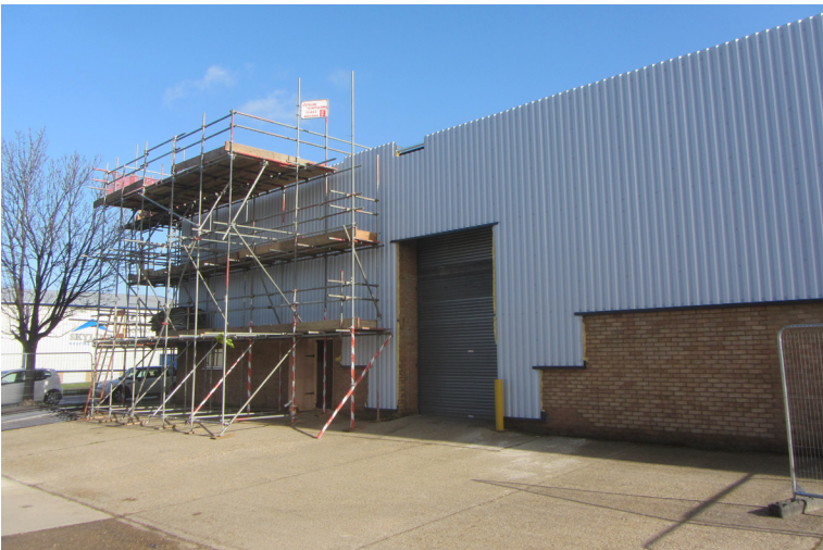
BUILDING MAINTENANCE & REPAIRS
